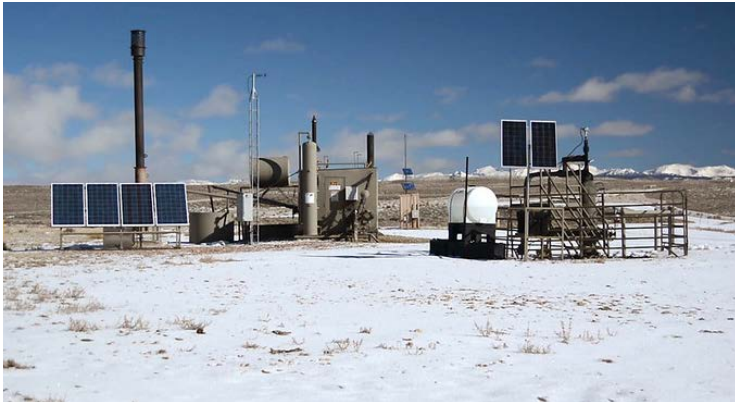
An example of a well-developed oil and gas facility; the burner stack is covered, solar power has replaced a noise generating engine, there is a closed-loop drilling system, and the overall footprint on the landscape is minimal. Photo: BLM Wyoming
