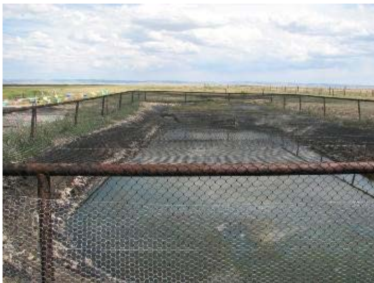
Pits created to capture oil waste, drilling fluids, and other liquid by products of oil and gas extraction can entrap or harm bats if they ingest compromised water and should be covered regardless of size. Photo: USFWS
