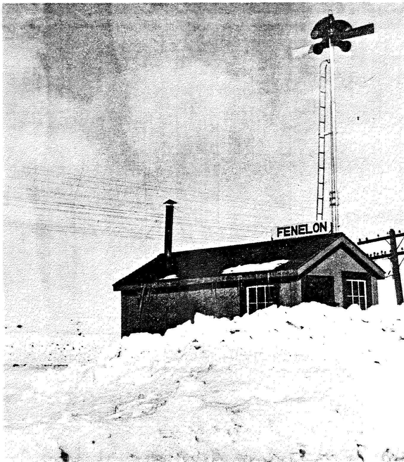
Southern Pacific signal station at Fenelon, Nevada, ca. 1940. Note relationship of semaphore, building, and telephone lines. (Photo courtesy of Churchill County Museum and Archive, Sharon L. Edaburn, Director.)
