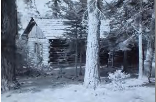
Railroad tie construction.
