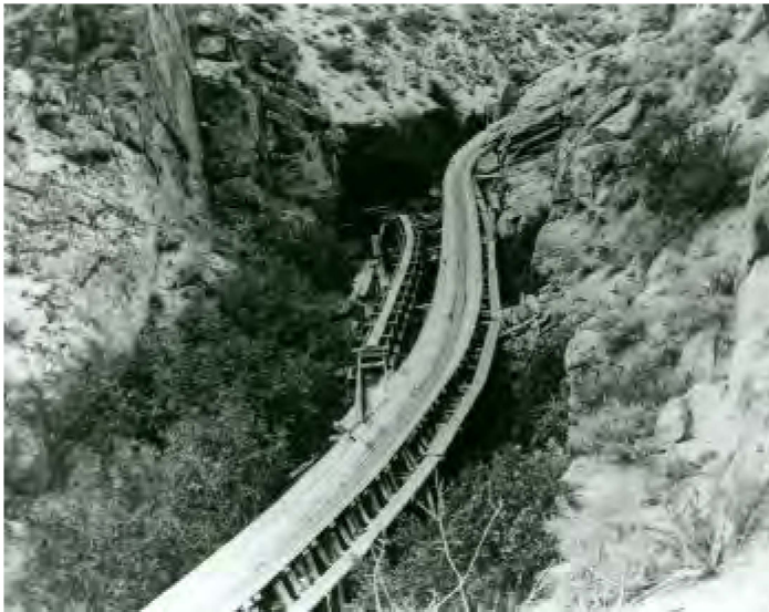
The Clear Creek Canyon flume, ca. 1890. The flume was 12 miles long, and linked Spooner Summit with the Virginia and Truckee Railroad yard about a mile south of Carson City.
