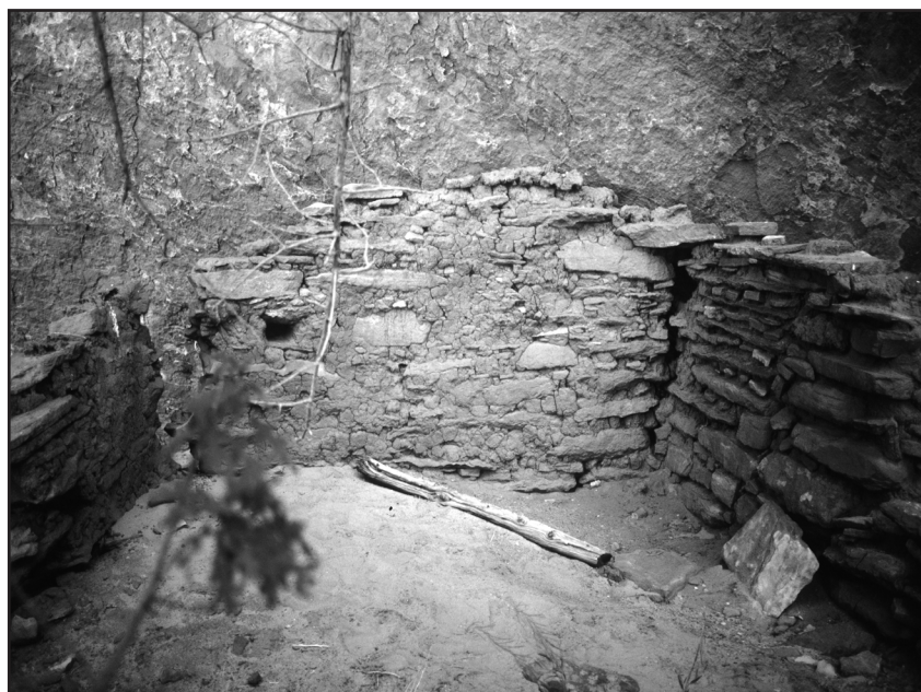
Figure 86. 42Ka1696 west room, note poorly bonded walls; 1970 photo (Kanab BLM files).
