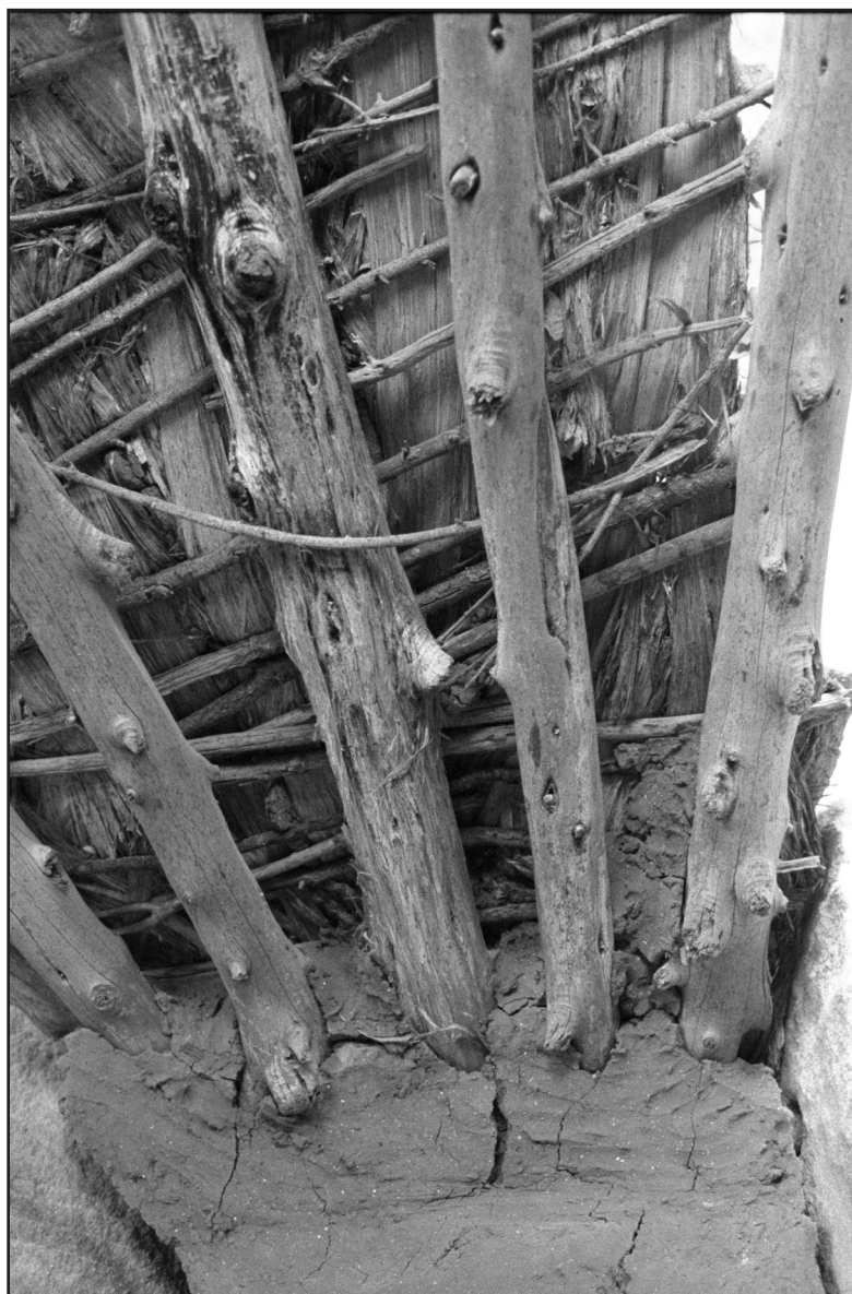
Figure 62. 42Ka1694, granary ceiling.
