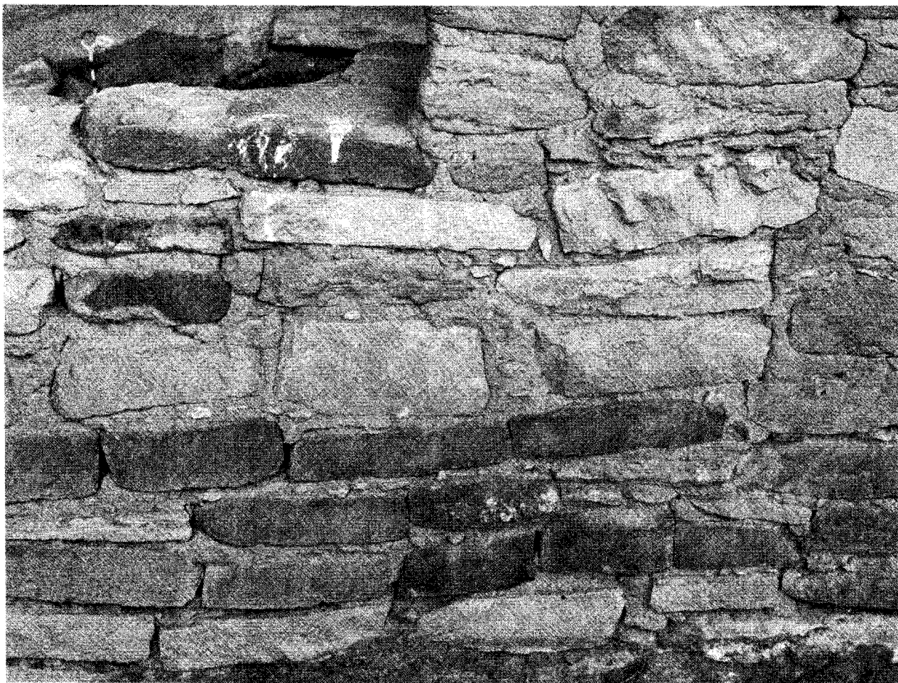
Figure 20 Closeup of the Masonry Construction of the Front Wall of Room 4
