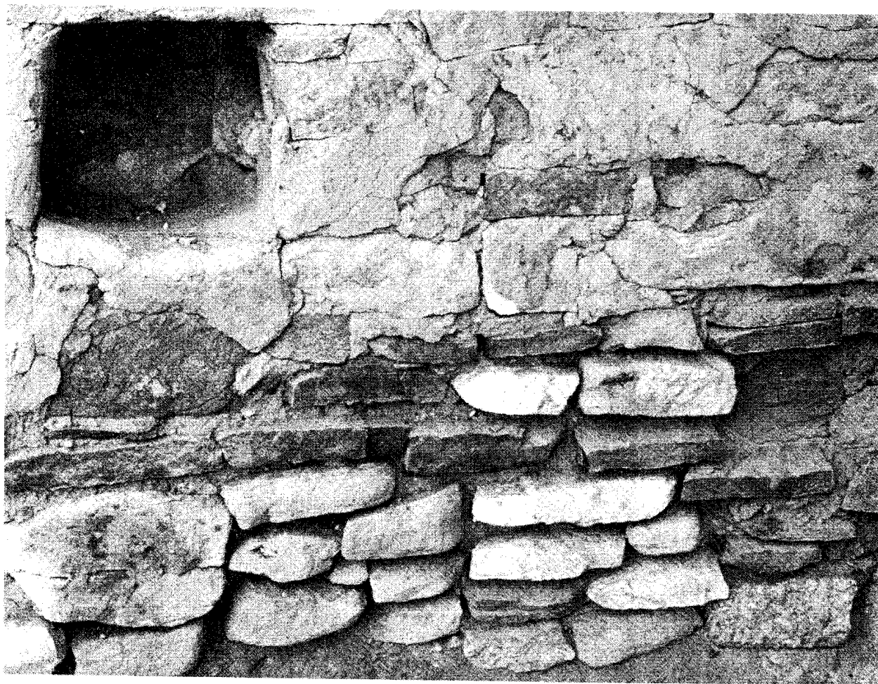
Figure 41 Closeup of the Rear Wall of the Kiva, Showing Masonry Detail and Wall Plaster (see Figure 26)
