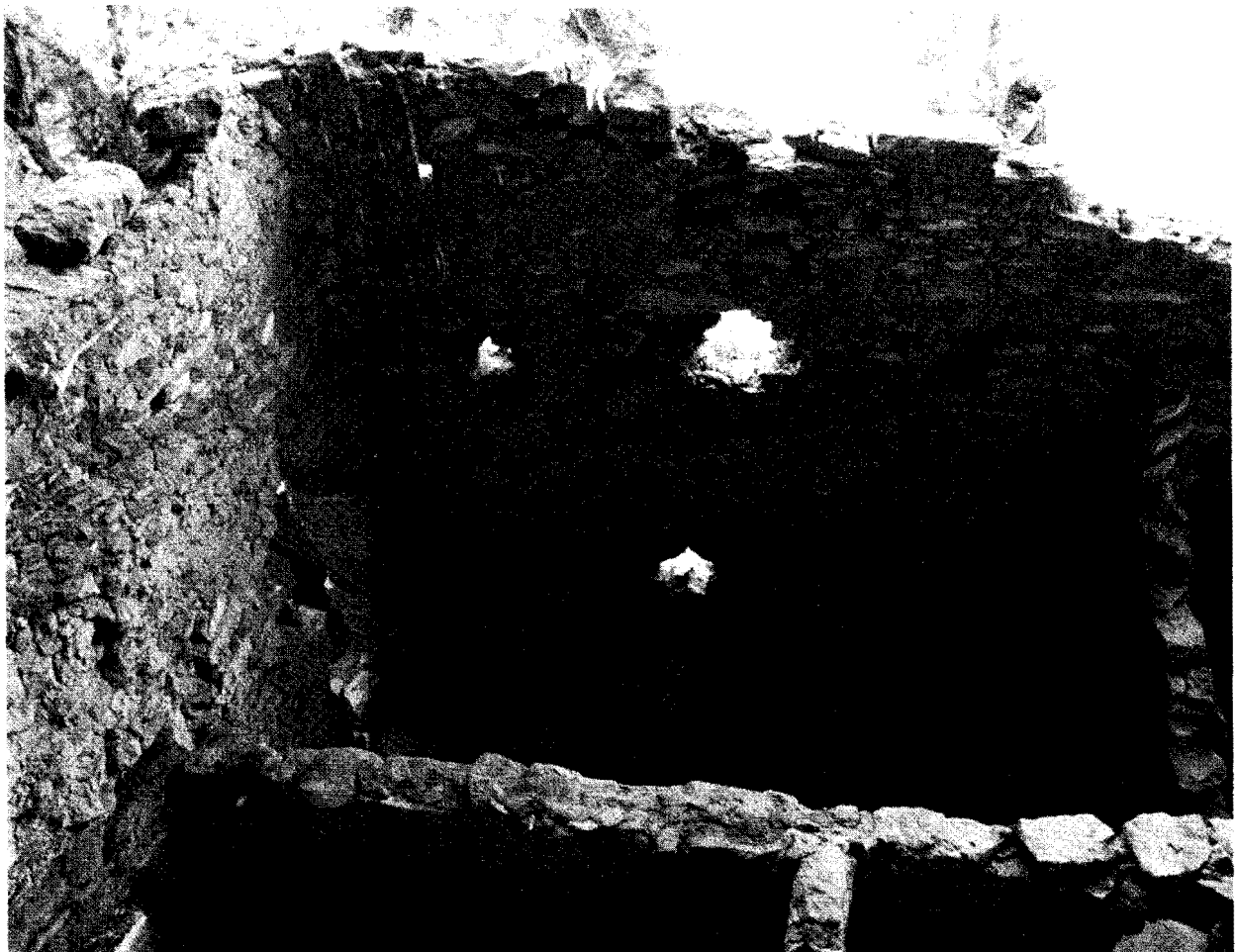
Figure 35 Room 9 from Rear of Shelter.
