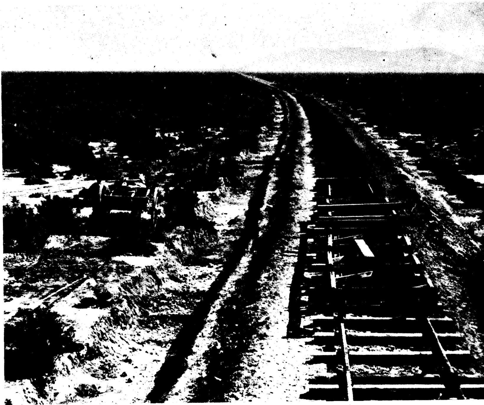
Figure 11: Track laying in the Utah desert (Southern Pacific, Alfred A. Hart Photograph).
