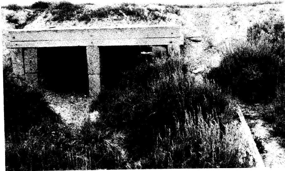
Figure 100: Dual wood box culvert (BLM photo)
