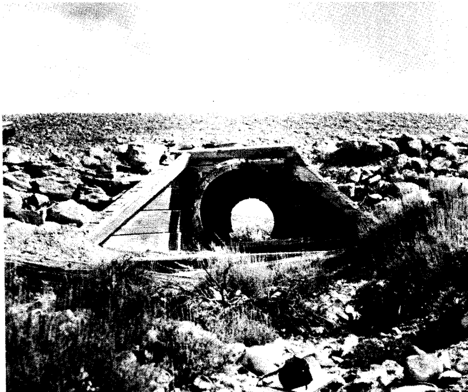
Figure 101: Wooden stave culvert with wing-walls, apron, and riprap. (BLM photo)
