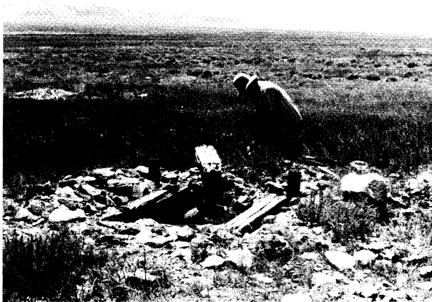
Figure 25: Outhouse foundation at Bovine (BLM photo)
