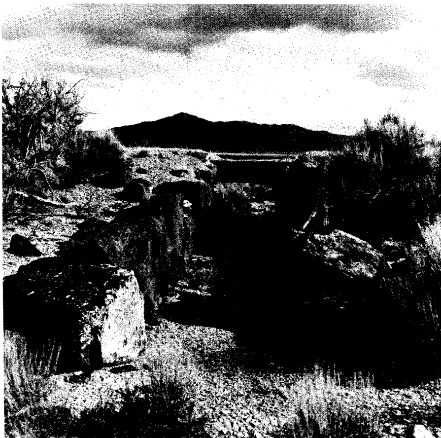
Figure 103: Open-deck stone culvert (BLM photo)
