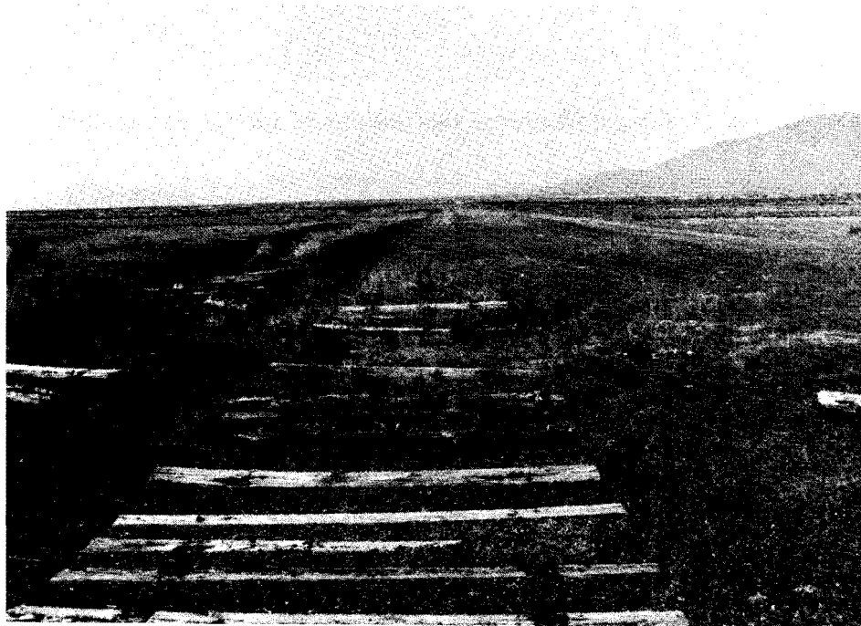
Figure 34: Terrace switchyard looking west (BLM photo)
