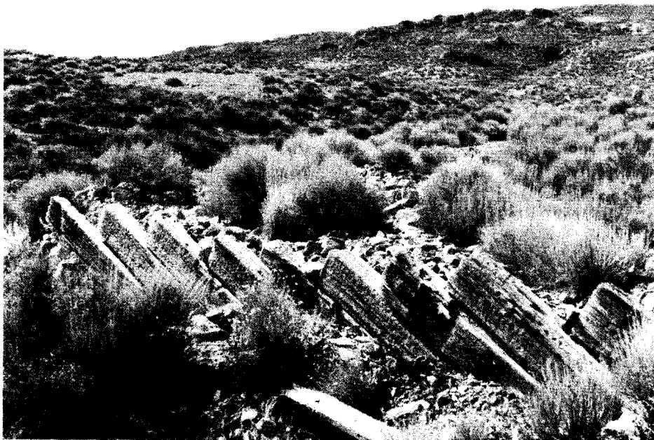
Figure 92: Railroad ties embedded in a wash channel to divert erosion away from the railroad grade. (BLM photo)
