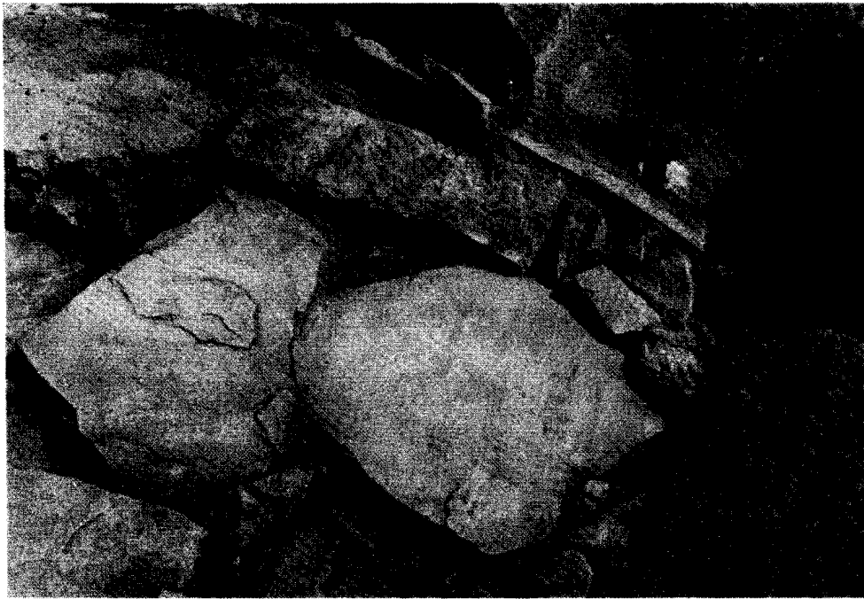
Figure 39. Room AI8, detail of tie of floor slabs to wall slabs.
