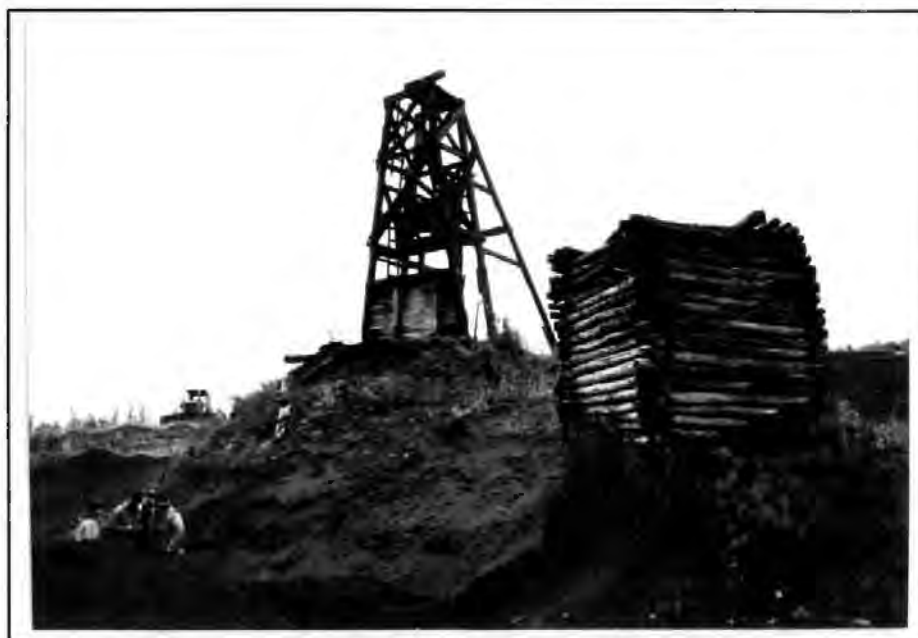
Figure 163. The Golden Horn Wood Framed Shaft (center) and Log Cribbed Shaft (right), 1993. The view is east.
