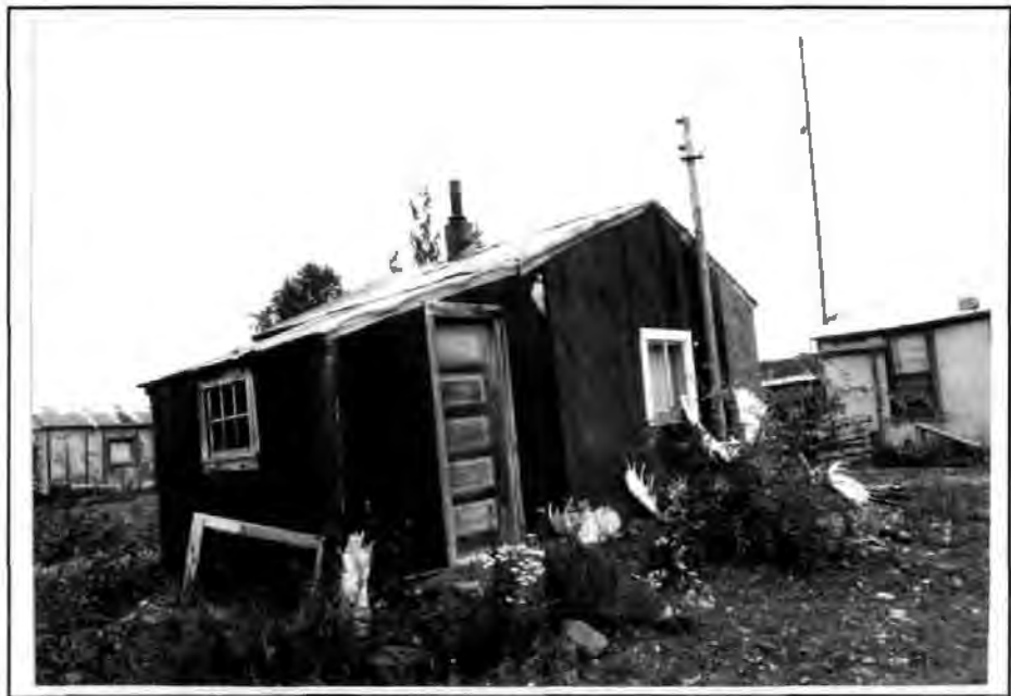
Figure 137. Bunkhouse #1, 1993. The view is looking southeast.
