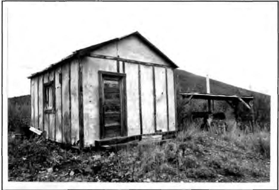
Figure 139. Bunkhouse #2, 1993. The view is looking northeast.
