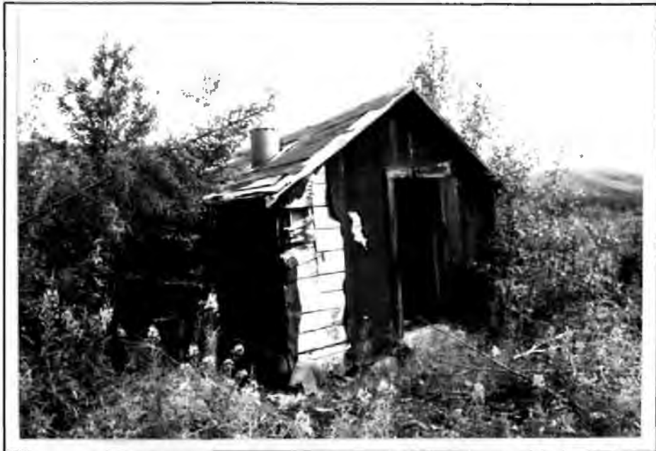
Figure 165. Small Bunkhouse, 1993. The view is looking southeast.
