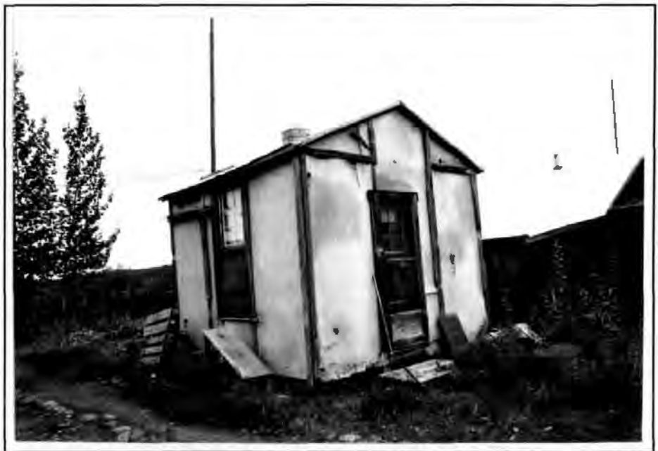
Figure 140. Bunkhouse #3, 1993. The view is looking southeast.
