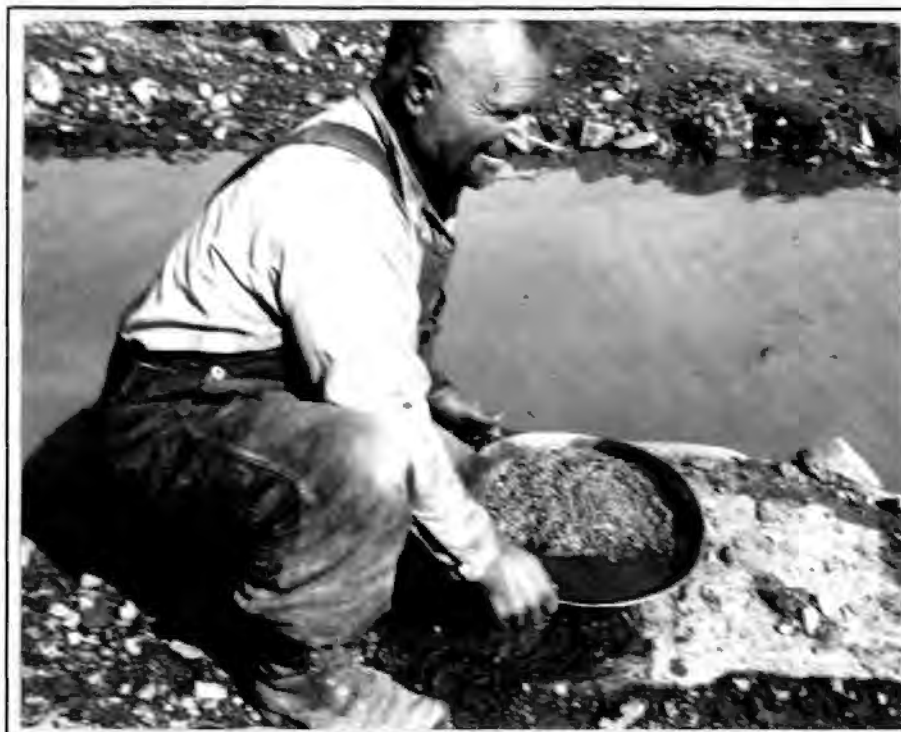
Figure 152. Peter Miscovich panning gold concentrates during a cleanup, 1935. Photo courtesy of Glen Barnett, Anchorage.
