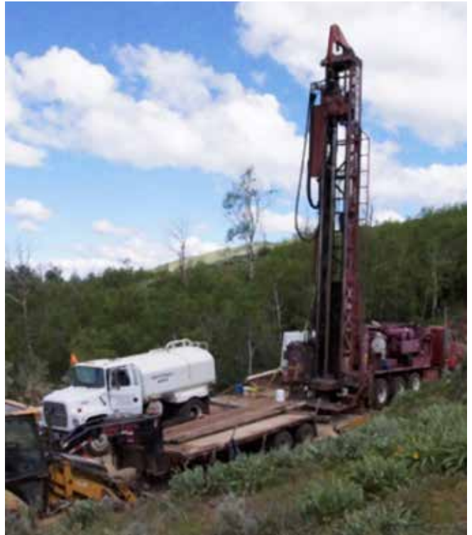
The BLM drills a groundwater monitoring well.
